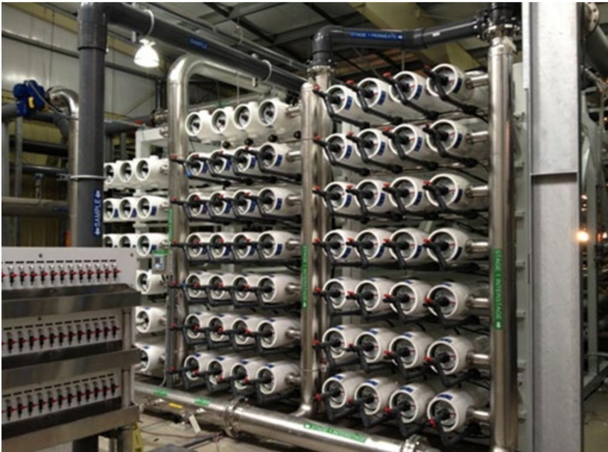
**Figure 4-1. RO Pressure Vessels and Sample Panel (bottom left) at YVWD to Allow Manual Conductivity Profiling.**
