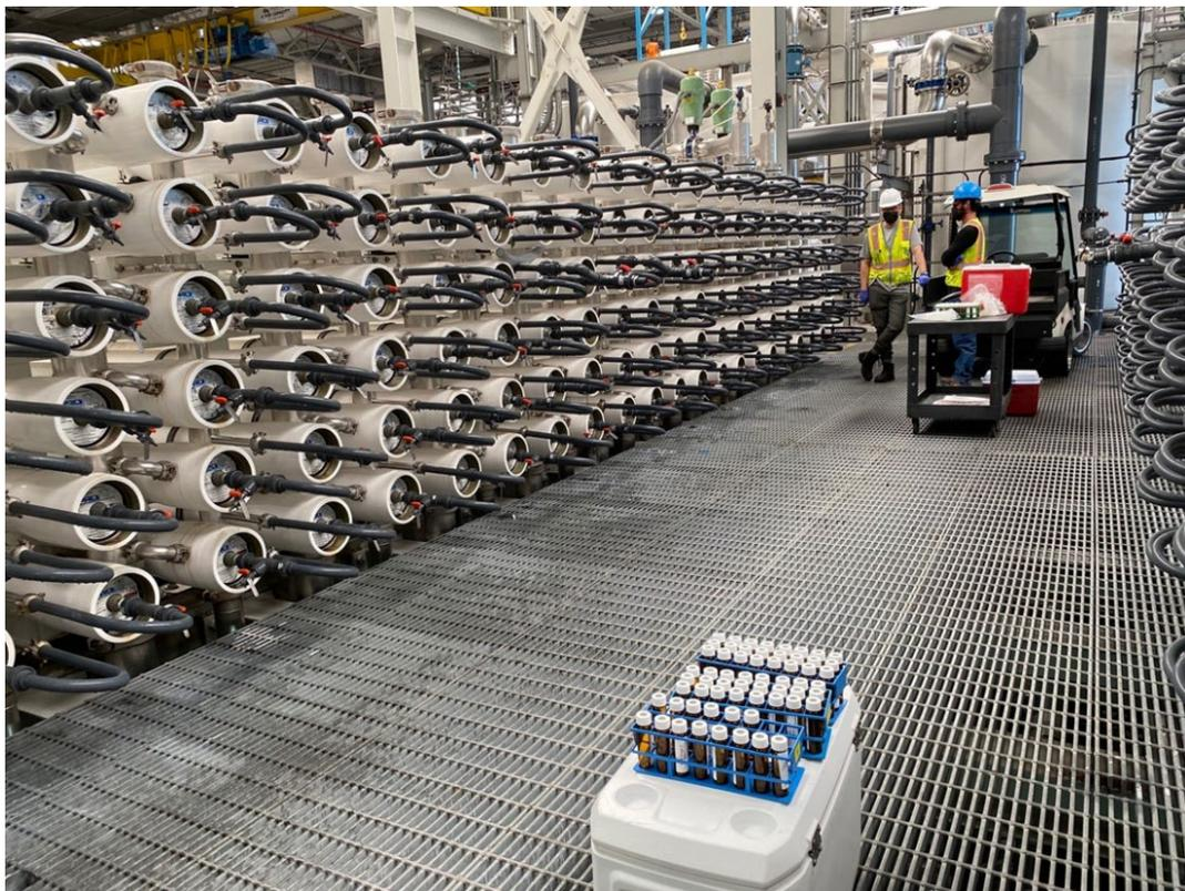
Figure 5-9. OCWD R&D Staff Await the Start of the Permeate Sampling for the GWRS 5 mgd RO Unit During the Uranine Dosing Experiment.
