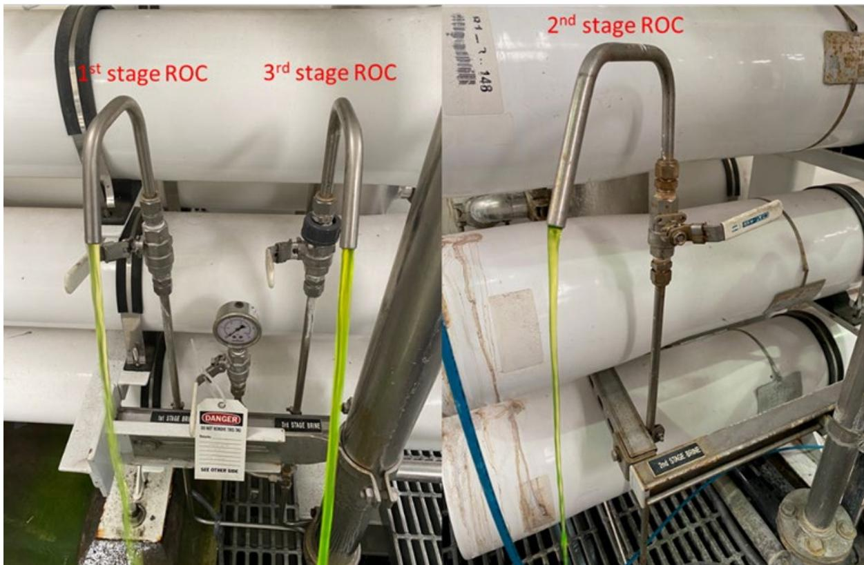
Figure 5-10. Photos of the RO Stage 1, 2, and 3 Concentrate Taps During Uranine Dosing Experiment.
