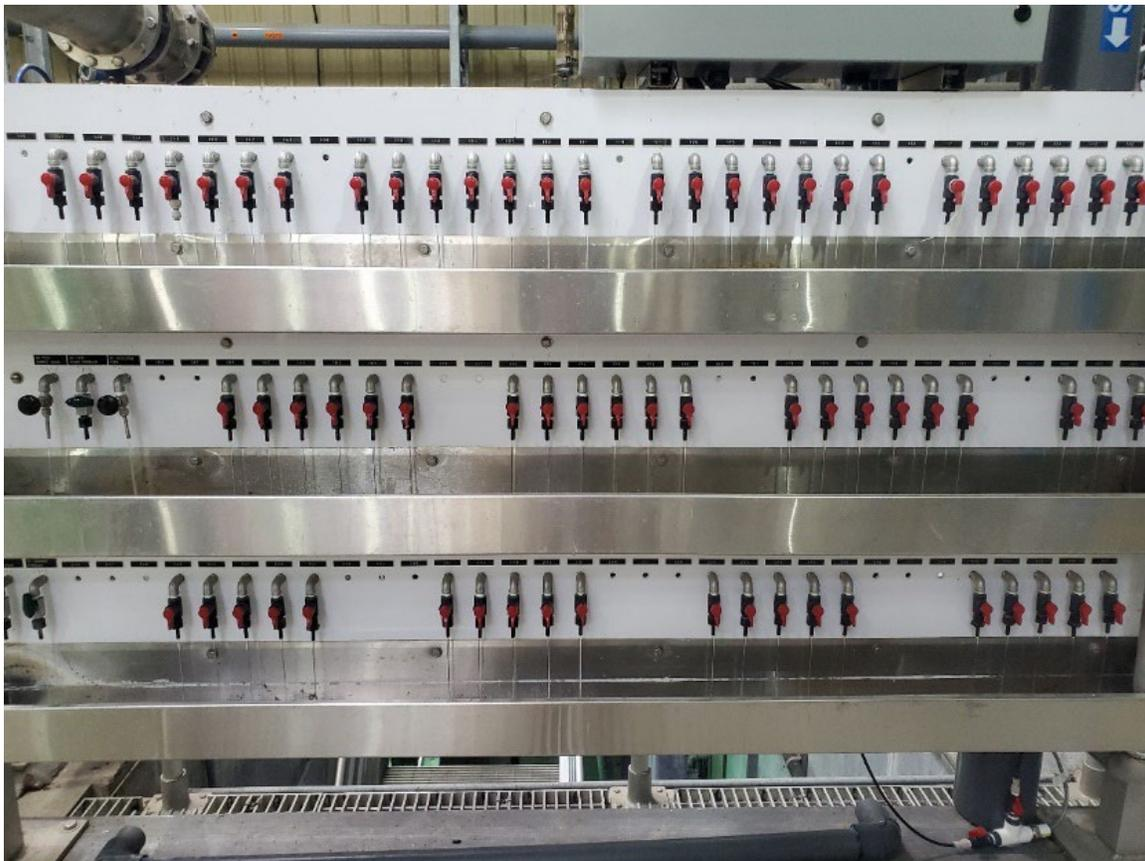
Figure 6-6. YVWD RO Sampling Ports Open for Flushing During Initial MS2 Dosing.
