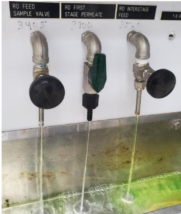
Figure 6-20. Streams from Sampling Ports at YVWD During Uranine Dosing.
