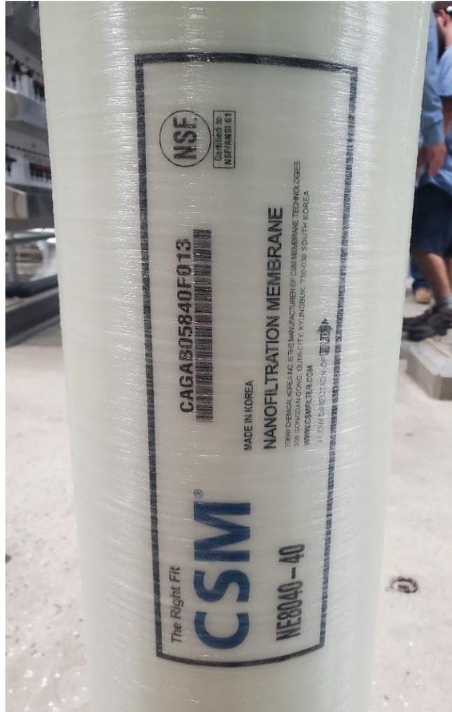
Figure 6-8. Nanofiltration Element Used to Substitute an RO Element at the Tail of Vessel 1-3-3.
