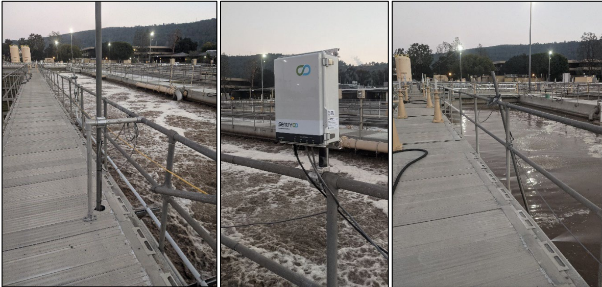
Figure 3-26. Sentry Probe in Primary Effluent (left), Communication Unit (middle), and Sentry Probe in an Anoxic Zone (right) of SJCEWRP.
