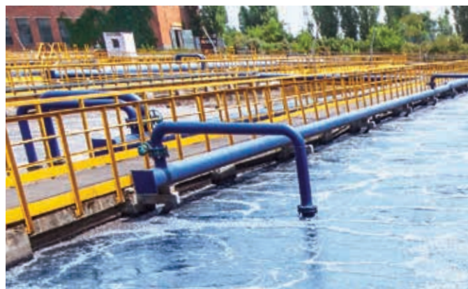
Figure 2. A wastewater treatment aeration tank is a source of N 2 O emissions, a potent GHG.
