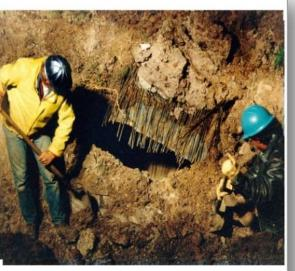
Dave Jones, left, and Bob Gonzales of the Otay yesterday morning near the Sweetwater Reservoir Water District help dig out a section of a main in Spring Valley. Two homes were damaged by pipeline of the San Diego Aqueduct that burst water when the 69-inch water line ruptured.
