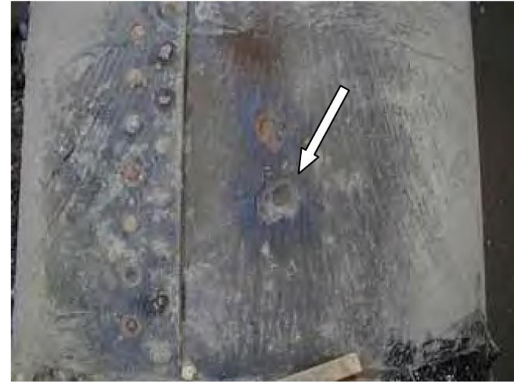
Figure 2.6. Exposed Cement Mortar Lining in 36-inch riveted steel pipeline. (Photo courtesy of Michael E. Grahek)
