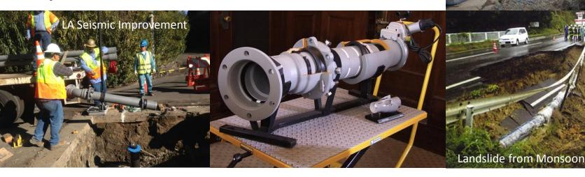
Examples of Kubota Earthquake Resistant Ductile Iron Pipe. Provide resilience for multiple hazards
