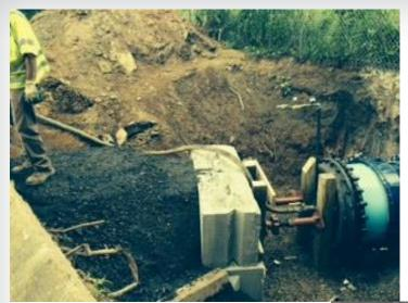
Restraint at connection and corrosion protection wrap
