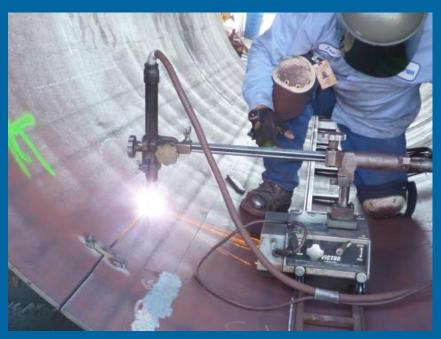
Overlapping the main longitudinal seam 3 inches, the backup bar is held with tack bars until it is skip welded from outside
