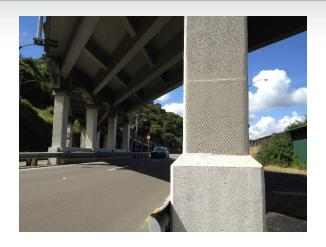
In 1996, Wellington's Aotea Quay Overbridge became the first bridge in New Zealand to be seismically strengthened with FRP composite materials.
