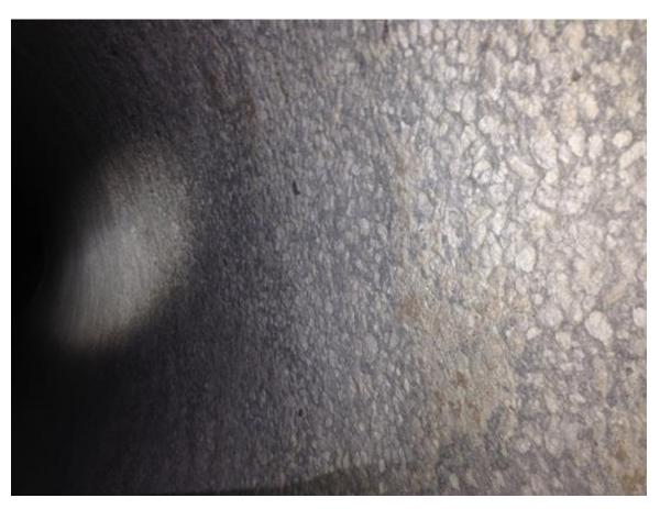
Prepared concrete substrate -54-inch PCCP
