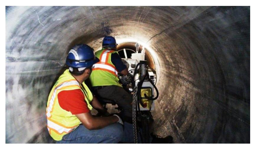
**Hybrid FRP System – Steel reinforcement installation**
