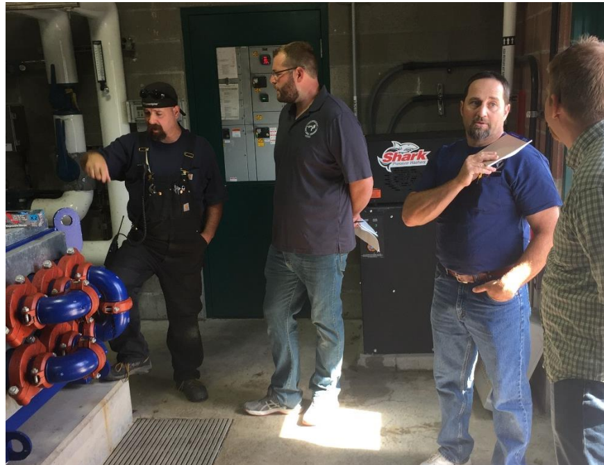
Figure 3: COB and CWS staff discuss lessons learned with the FOG Receiving Station at the Durham Advanced Wastewater Treatment Facility
