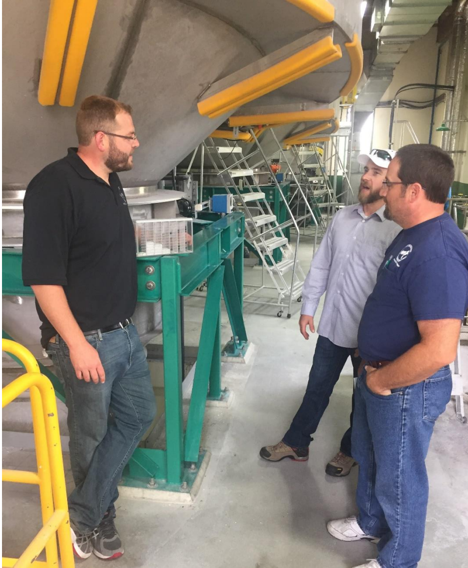
Figure 2: Staff discuss struvite harvesting technology during a tour of the Ostara Pearl System at the Durham Advanced Wastewater Treatment Facility
