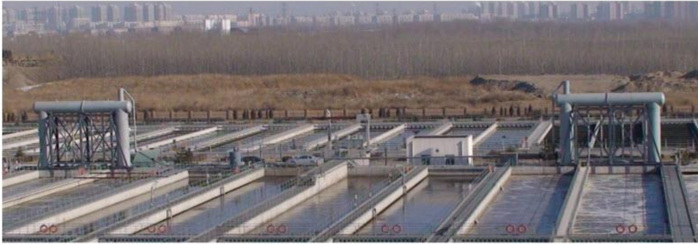
Figure 4: Qinghe WWTP, Section 2, North Train – overall view of bioreactors, secondary clarifiers and the vacuum towers
