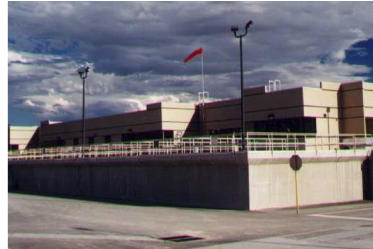
Contact Clarifier – Filter converted to Direct Filtration
