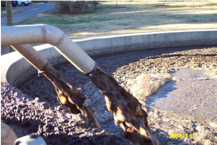
Reduced Sludge Production Process Operate as Aerobic Digester
