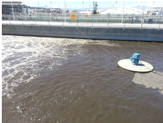
Surface flow from Aerobic to Anoxic Zone
