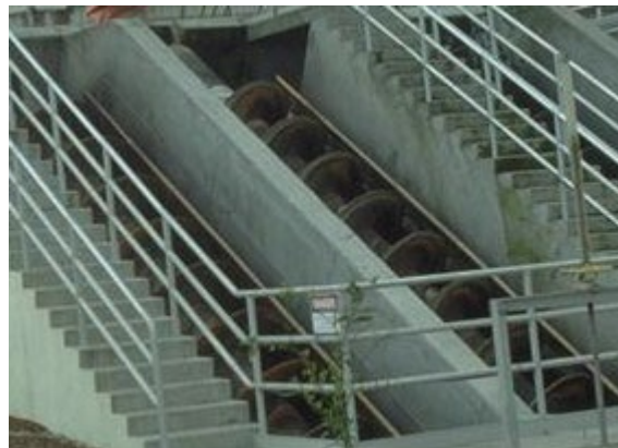
Screw pump for RAS return
