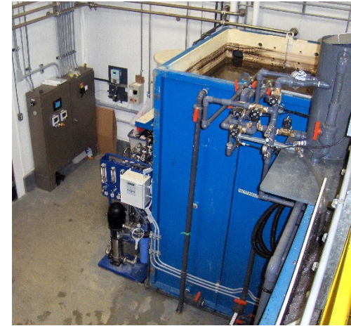
Membrane Bioreactor: First system in the world to upgrade effluent water for reuse in production in compliance with Federal Food Regulations in beverage manufacturing
