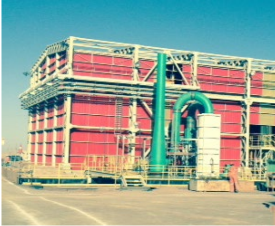
Acid Mist Scrubber: Chilean mining operation
