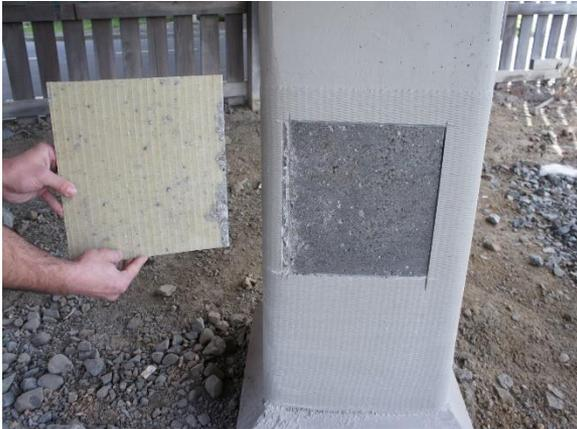
In 2013, a panel was carefully abstracted and tested at a certified laboratory
