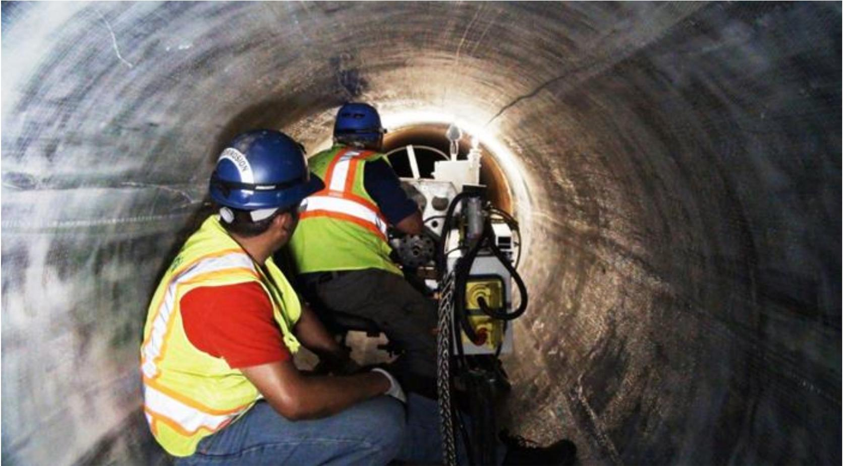
**Hybrid FRP System – Steel reinforcement installation**
