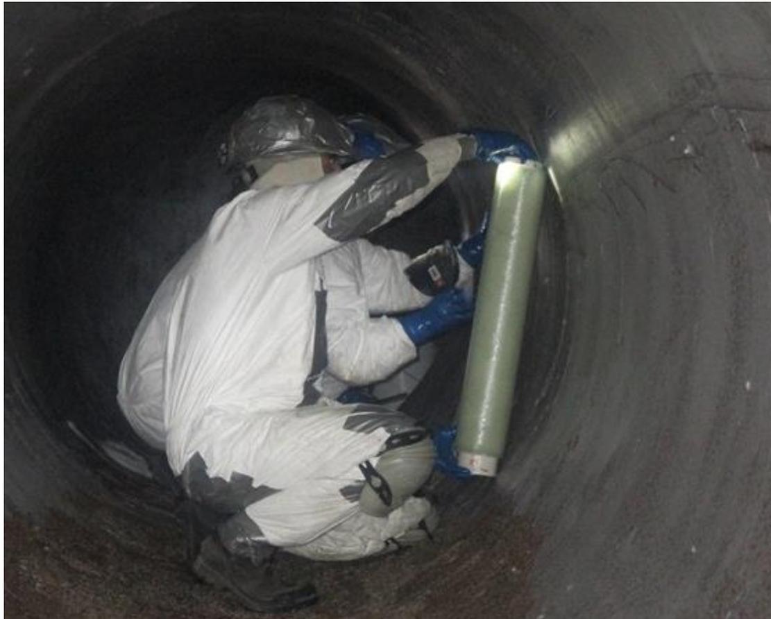
**Installation of longitudinal layer of fiber reinforced polymer**
