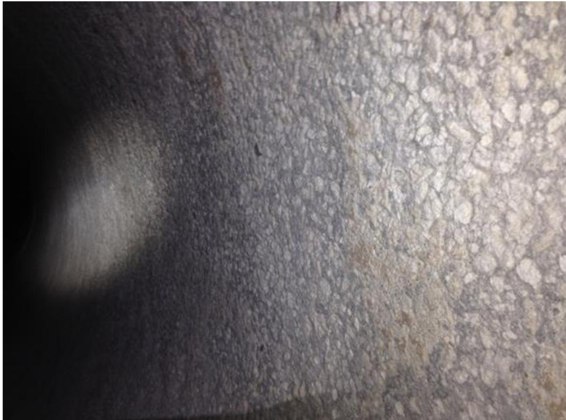
**Prepared concrete substrate –54-inch PCCP**
