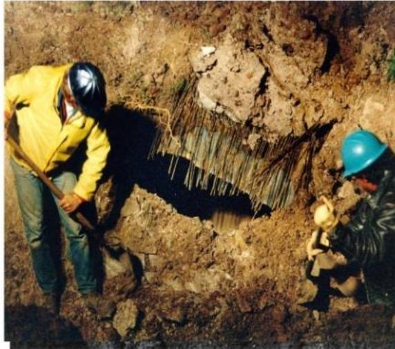
Dave Jones, left, and Bob Gonzales of the Otay Water District help dig out a section of a main pipeline of the San Diego Aqueduct that burst yesterday morning near the Sweetwater Reservoir in Spring Valley. Two homes were damaged by water when the 69-inch waterline ruptured.
