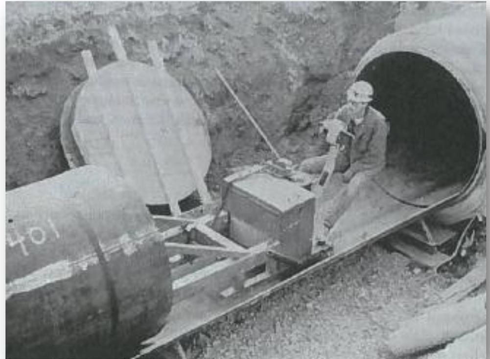
Steel Liners Inserted into Pipe (1982)
