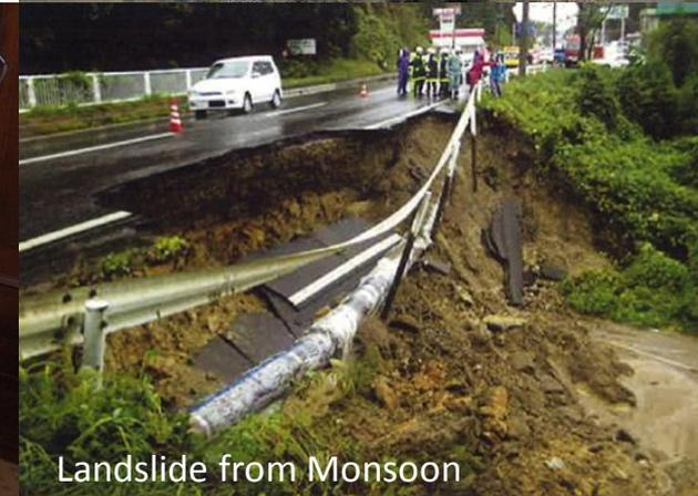
Examples of Kubota Earthquake Resistant Ductile Iron Pipe. Provide resilience for multiple hazards
