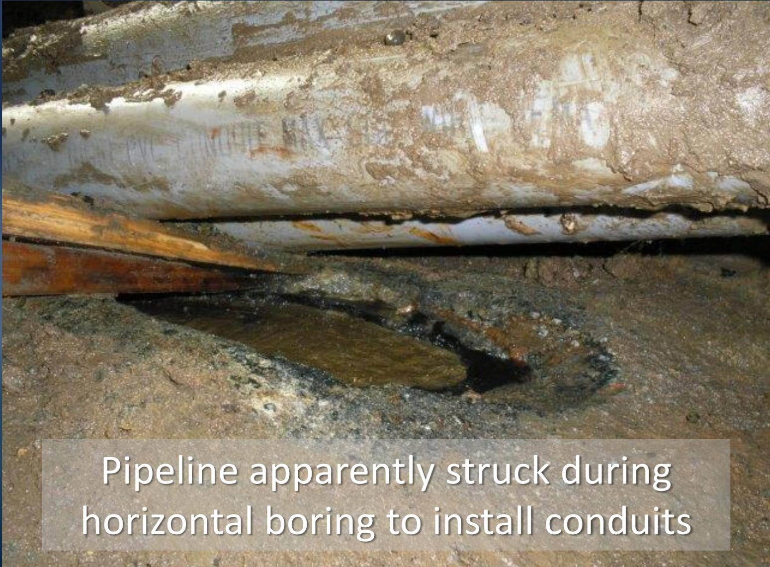
Pipeline apparently struck during horizontal boring to install conduits
