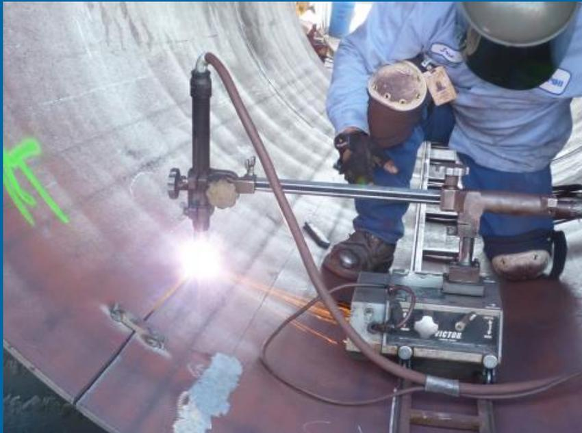
Overlapping the main longitudinal seam 3 inches, the backup bar is held with tack bars until it is skip welded from outside
