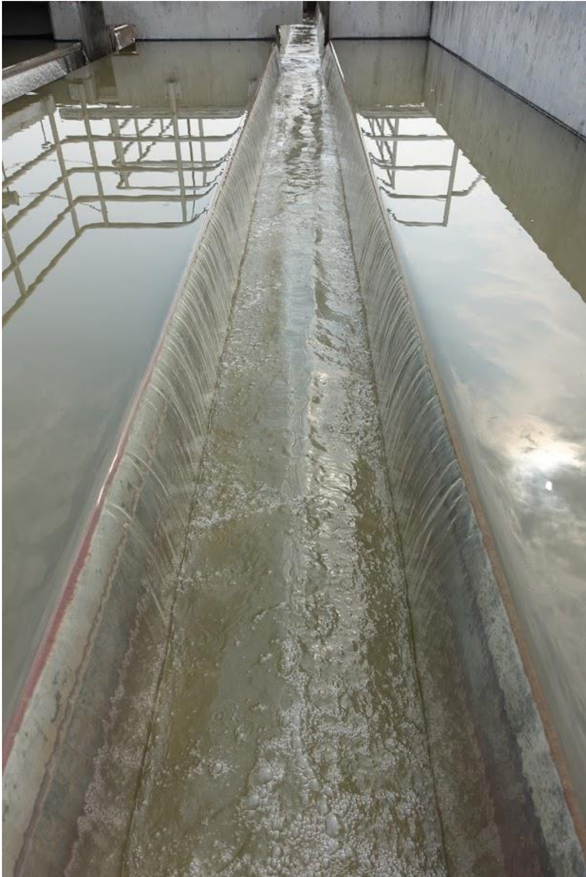
Primary effluent water spilling over straight weirs (KalisPELL)
