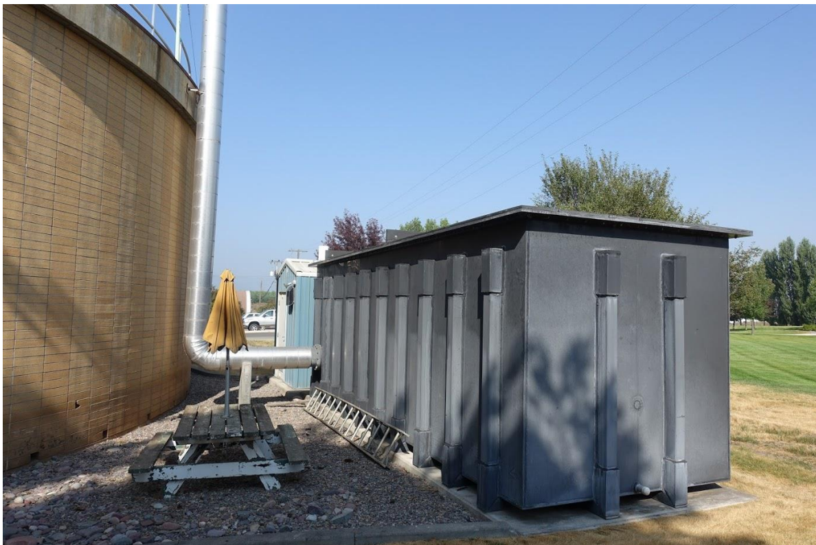
Exhaust air from the fermenter is routed through a woodchip biofilter for effective odor control (Missoula)
