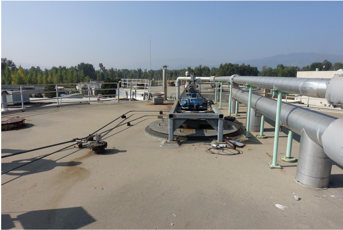
Roof and sludge mechanism of the single stage primary sludge fermentation tank (Missoula)
