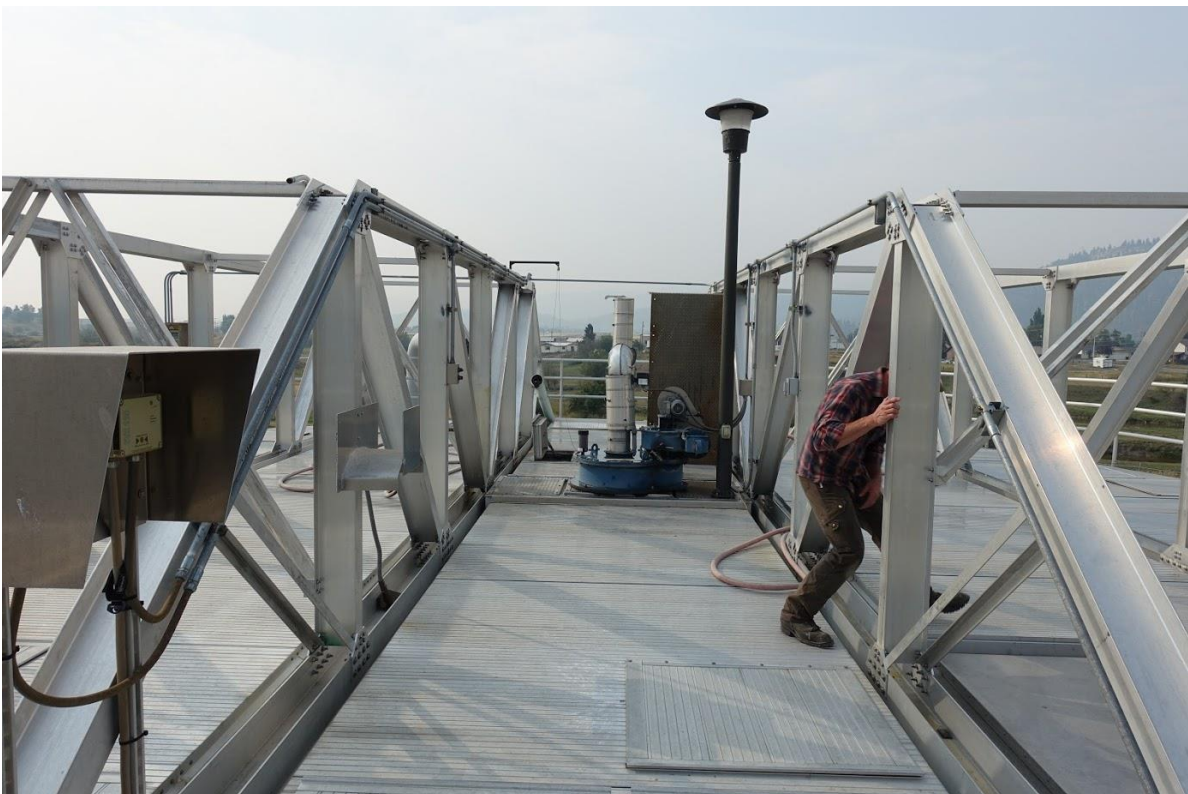
Fermenter cover and sludge mechanism (Kalispell)
