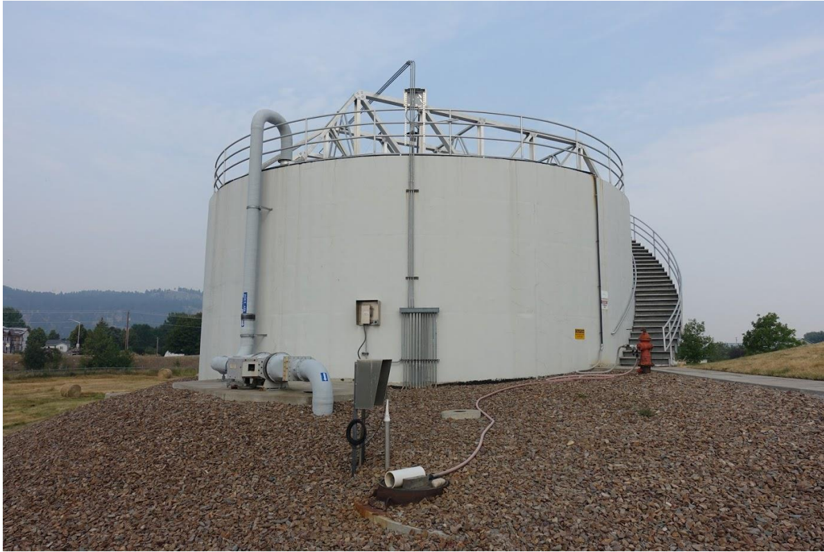
Single stage primary sludge fermenter (Kalispell)
